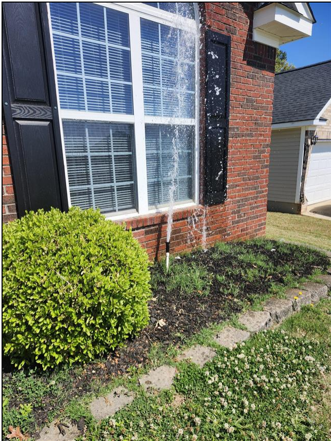
11.1 Item 1 (Picture) Sprinkler head at front of home is broken.
